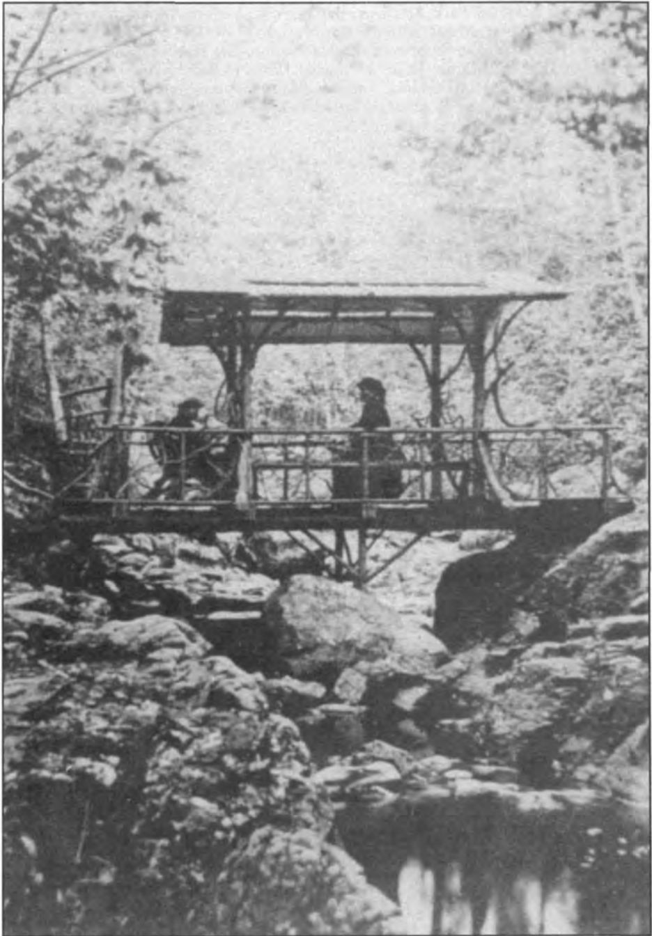
Figure 1. A footbridge over Duck Brook indicates the influence of the picturesque style on the early development of the trail system, ca. 1870. Photographer unknown. Courtesy Acadia National Park Archives.
