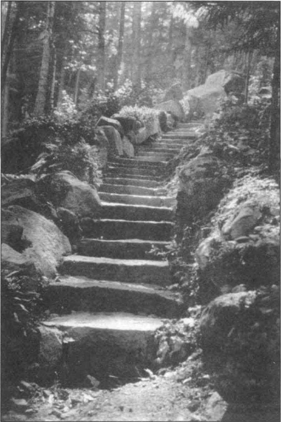
Figure 4. Stone staircase on the Emery Path, ca. 1916. Photographer unknown. Courtesy Acadia National Park Archives.
